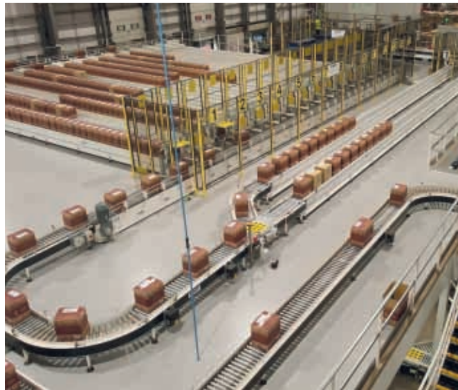
Accumulation and handling of the cases has moved to a new mezzanine
