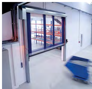
All goods movement needs are met
